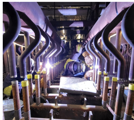
PIPING REPAIR/REPLACEMENT.
